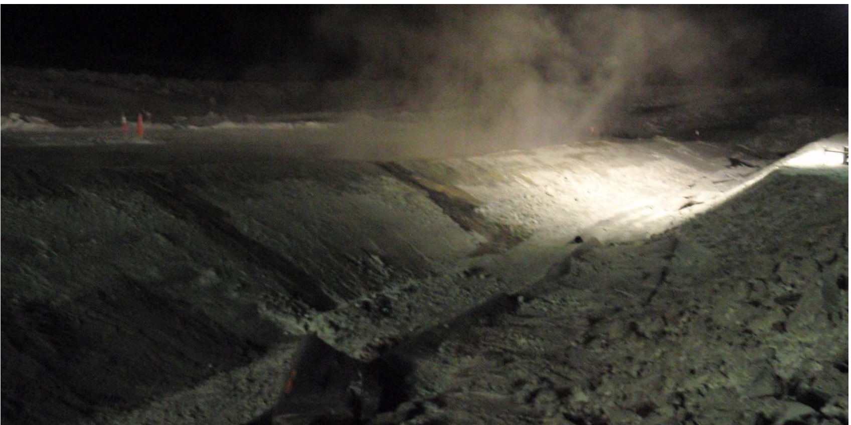
Photo 16: ~N view of upstream core slope. Note areas where water ponded and seeped/ discharged down the upstream slope. The ice on the slope in these areas is expected to be scraped down along with the areas of minor water erosion. Some additional FCM is expected to be required near the upstream crest in these areas to bring the crest to the design lines / limit.
