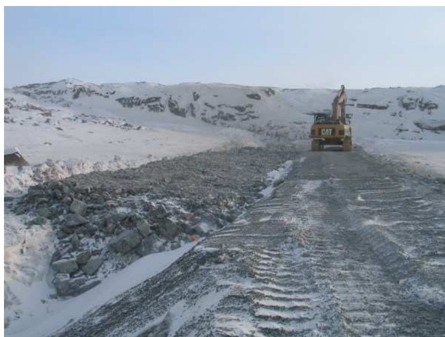
Photo 11: Excavator continuing with ROQ placement at the berm
