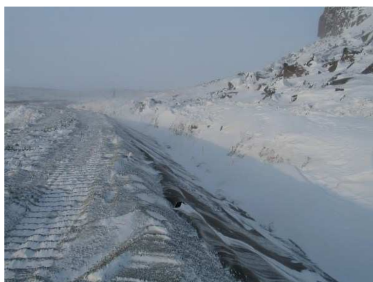
Photo 12: Snow in key trench that needs to be removed before any further work can be done.
