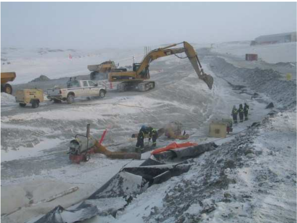
Photo 7: Excavator clearing snow at bottom of core. Labourers ready to blow snow. Labourers in foreground working with frost fighters.
