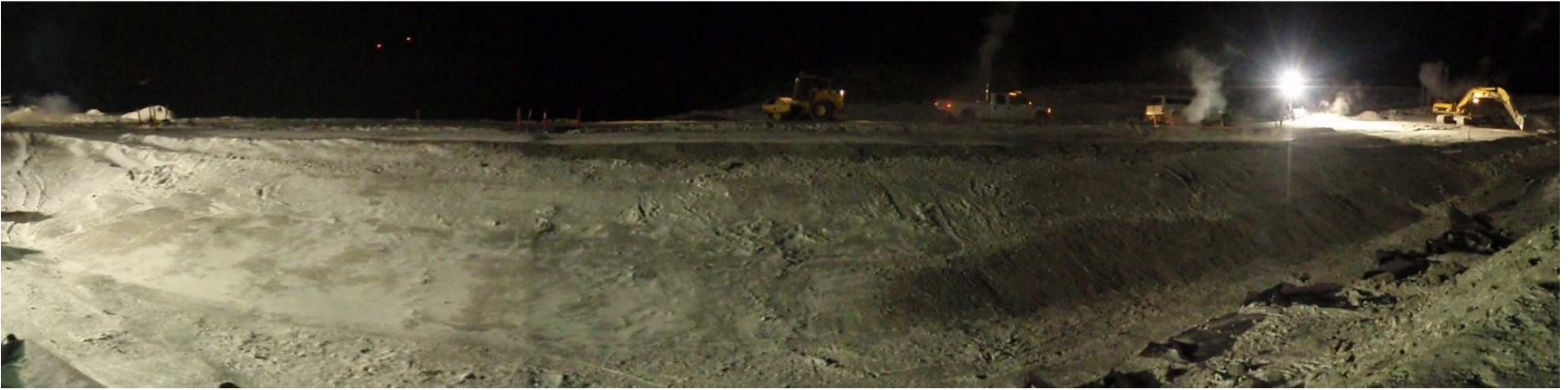
Photo 13: Stitched panoramic view of the upstream dam slope. Taking looking ~NNE from the dam shell around station 0+90. Note the dark patch in the bottom right of the picture that shows the area where dayshift placed FCM to remove the lower 'steps' in the upstream slope.
