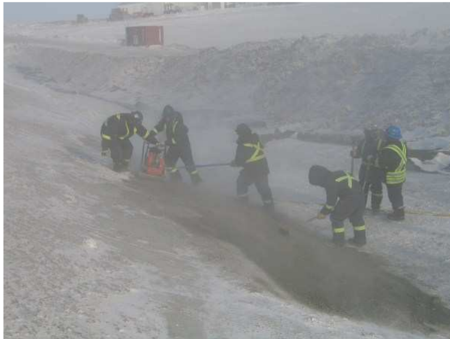
Photo 9: Raking and compaction at bottom of slope.
